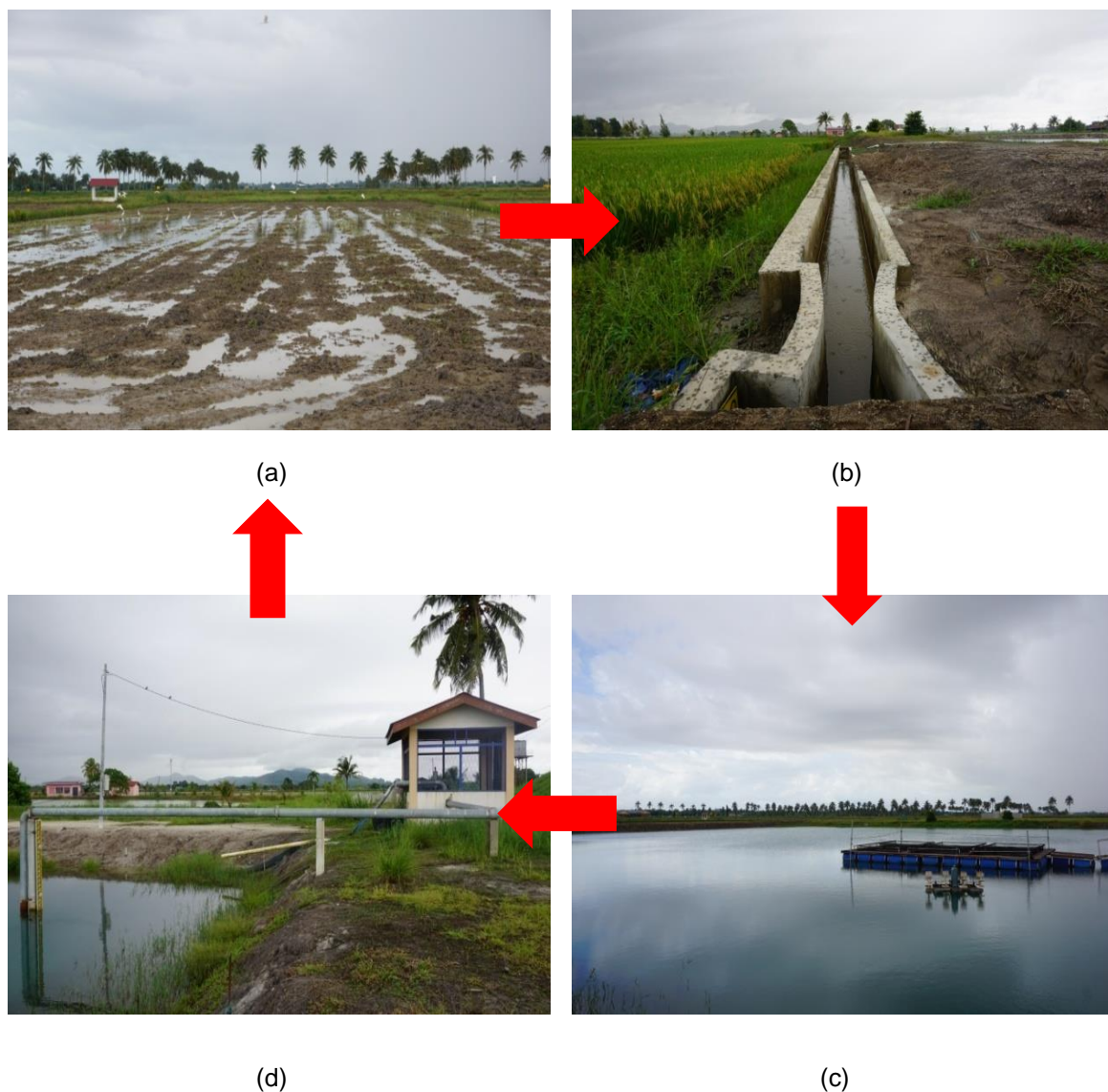
Figure 1. Schematic flow of water recycling system (a) Field water catchment area and irrigated water; (b) Perimeter drain convey water to the recycle pond; (c) Water collected in recycle pond; (d) Pump house facilities for a pipeline irrigation system.
